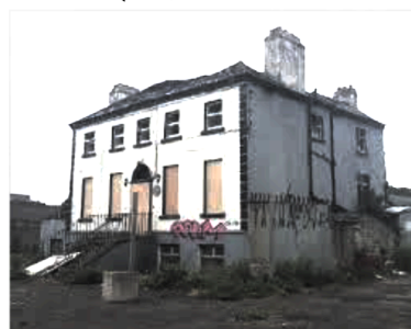
Glebe House, Crumlin Village
