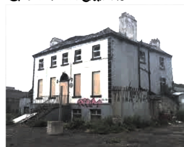
Glebe house, Crumlin
