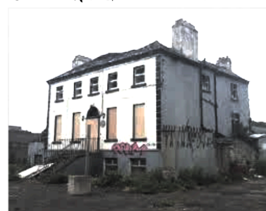
Glebe House, Crumlin Village
